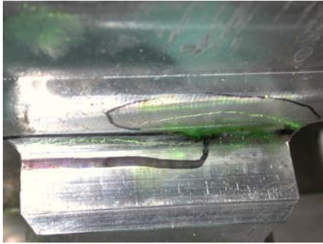
Figure 7a. A close-up optical image of part of the object shown in Fig. 6 showing penetrant seeping from a crack (Green).
