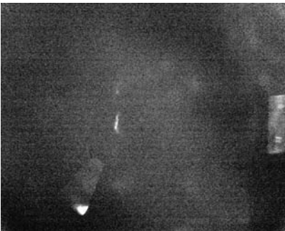
Figure 10a. An IR image taken shortly after the sonic excitation was turned on. There are two cracks extending from a rivet located on the left of the image center, a longer one underneath, and a shorter one above.
